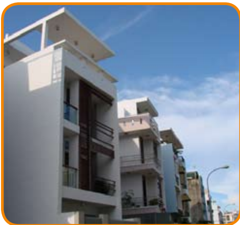
Examples of constructive shading in town houses and apartments (Source: Waibel, 2011; Schwede, 2010)
