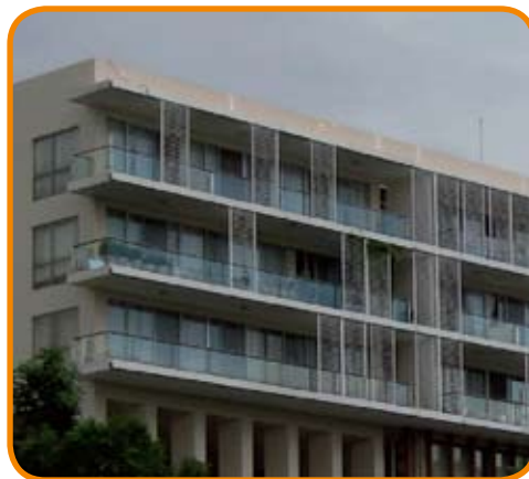
Examples of constructive shading in town houses and apartments (Source: Waibel, 2011; Schwede, 2010)
