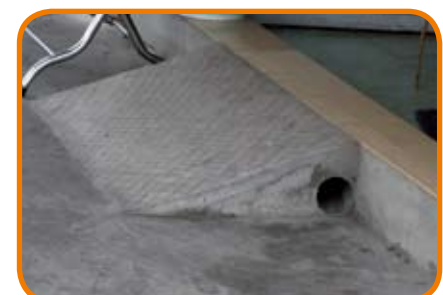
Tubes to allow the water to flow off (Source: Hang 2010; Waibel 2011)
