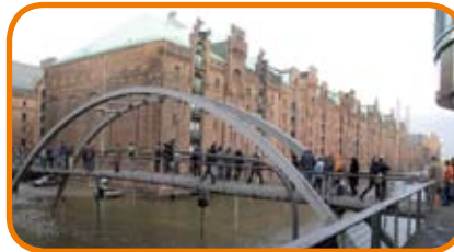
Permanent emergency service ways
