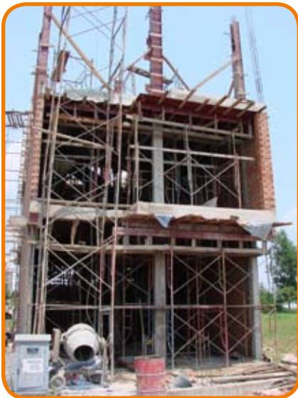
Town house under construction, light brick is used as insulation (Source: Waibel 2010)
