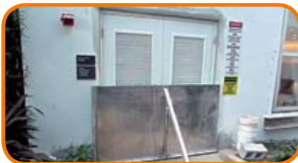
Permanent and mobile sealing of openings (Source: ICPR 2002/www.floodpanel.com)
