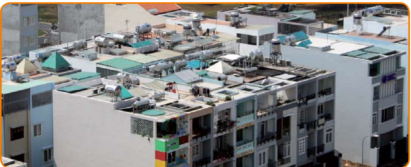
Examples of solar water heater use in HCMC (Source: Cüce 2011)
